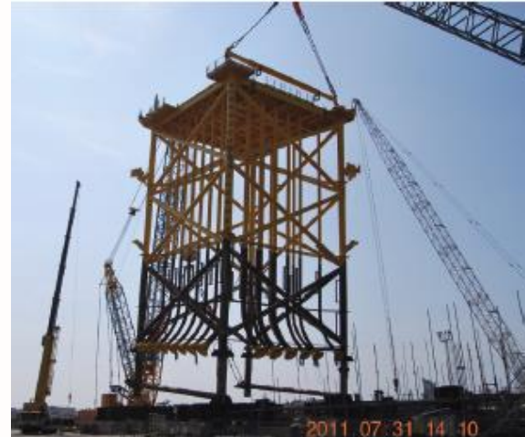
Source: OWEC (C-Power – 325 MW - 2,000 MT)
