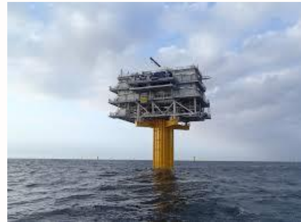
Source: Northwind (216 MW – 1,200 MT)
